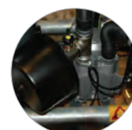
Inlet blower filters
